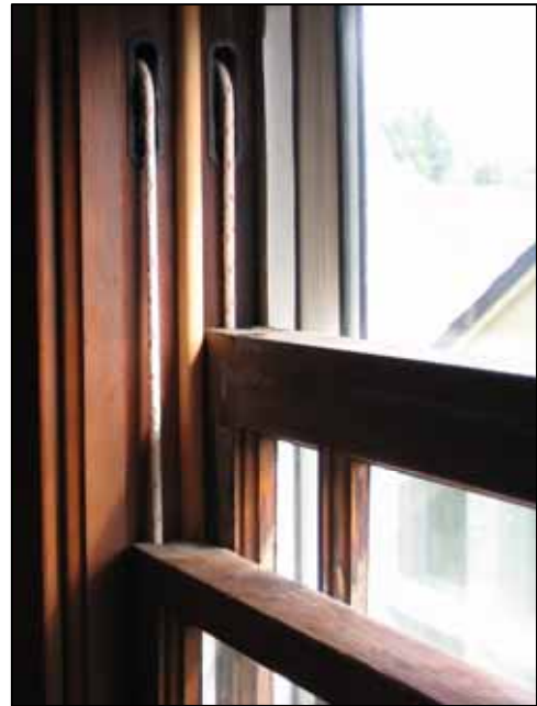
Unpainted jambs decrease friction and allow window sashes to open and close more easily.
